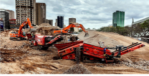
Renico Quarrying & Crushing equipment in operation.
